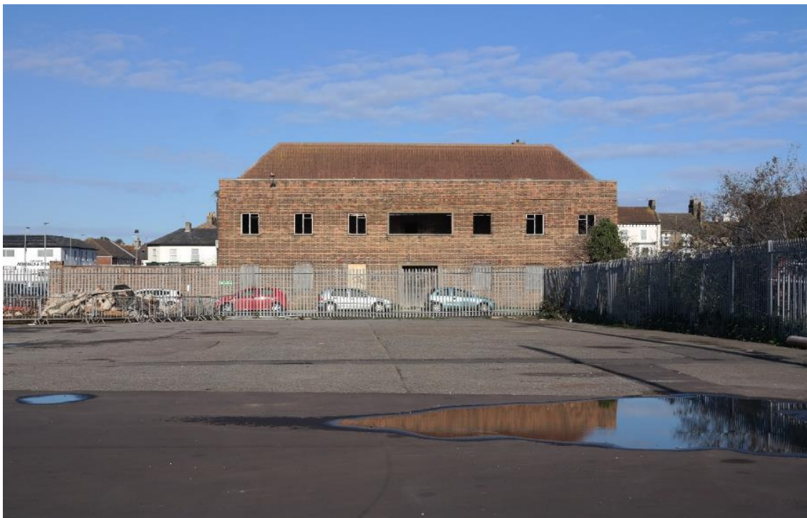
Plate 9-13 - Goods Office for Freight Yard, Commercial Road
