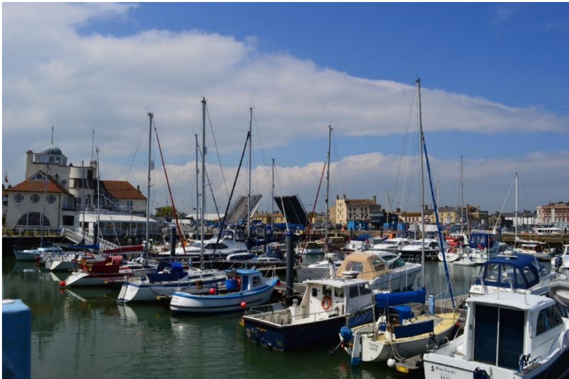
Plate 10-2 – View across the marina towards the A47 Bascule Bridge and the entrance to Lake Lothing
