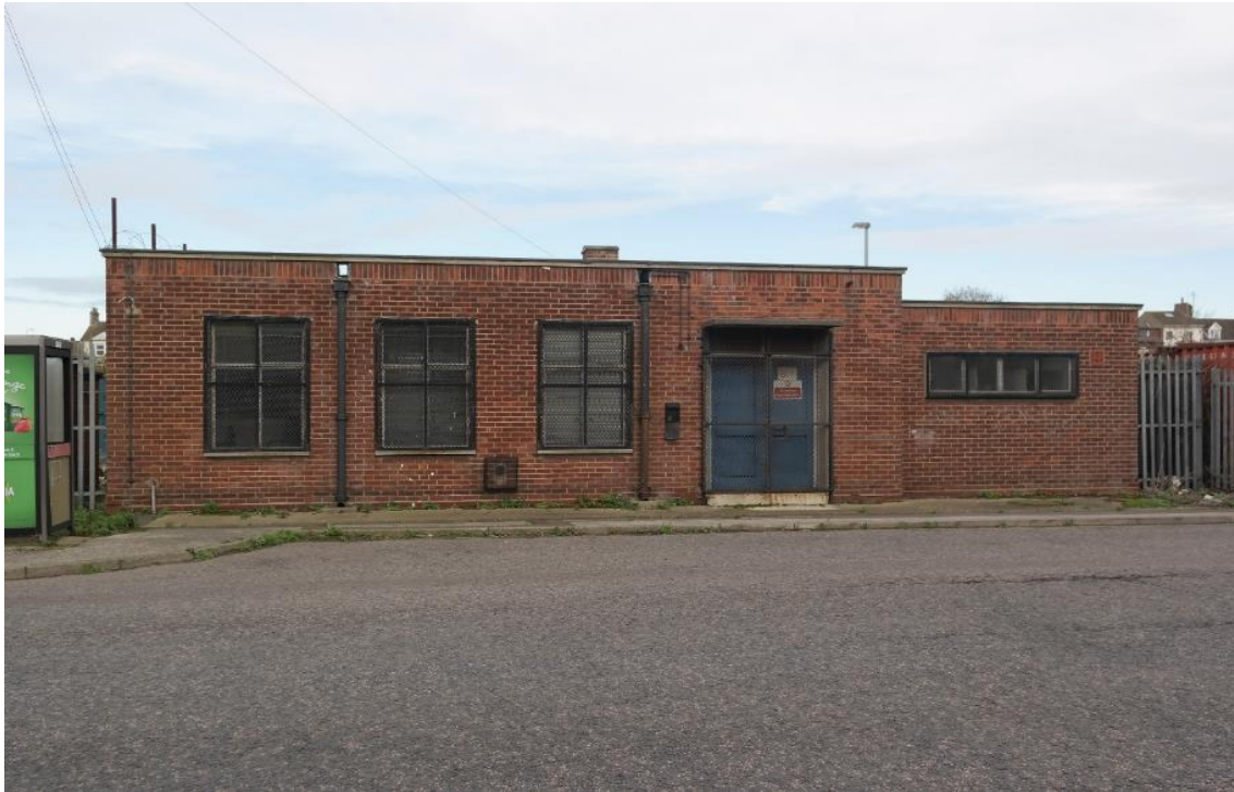
Plate 9-14 – Freight Yard Building, Commercial Road
